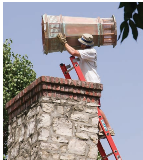
Installing a traditional chimney pot.
