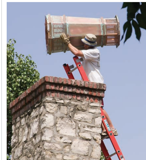
Installing a traditional chimney pot.
